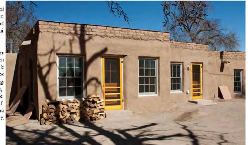
At Ohkay Owingeh, new and renovated homes in the pueblo incorporate locally sourced materials and traditional construction techniques like adobe and mud plaster, supporting local labor and strengthening settlement patterns and cultural activities that are centuries old. Katie Russell Photography
